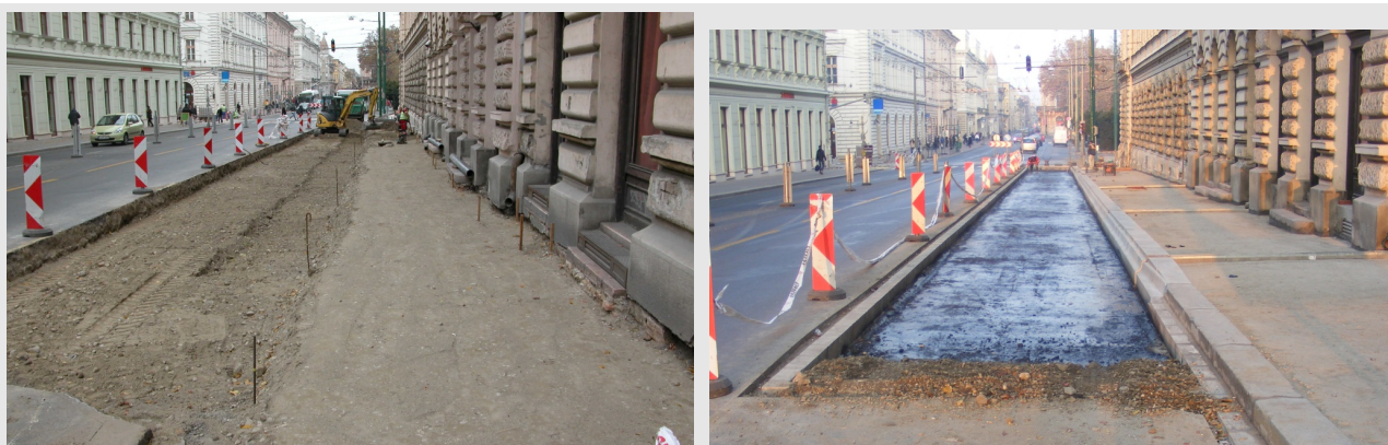
Two stages of the reconstruction of the trolleybus stop. The neighboring lane were mostly kept free for traffic.
