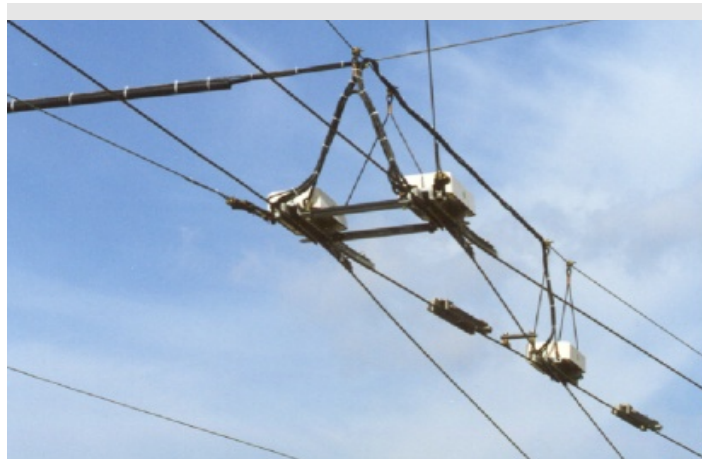
Modern strained trolleybus symmetric 10° turnout
