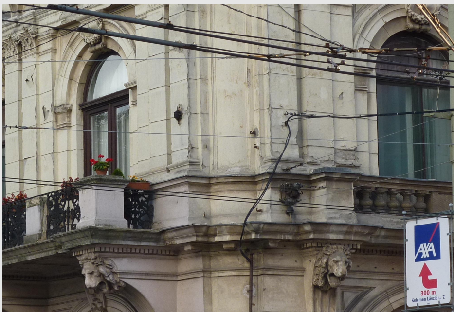
Different used and unused hooks of the trolleybus catenary on a private building before the project. One can spot a historic unused one, which belonged since 1909 to the ancient tram
