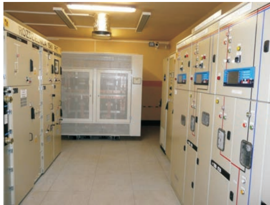
Fig. 4.14. Interior of a single unit traction substation (Gdynia, Poland)
