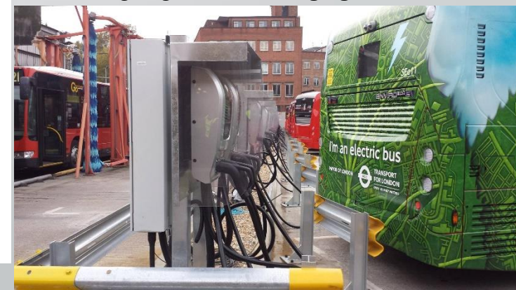
Waterloo garage 3,6 MW charging infra (46 buses)
