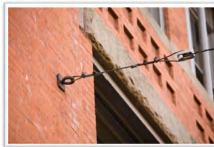
Exhibit 5-8. Trolley Bus Wire Anchored to Historic Structures
