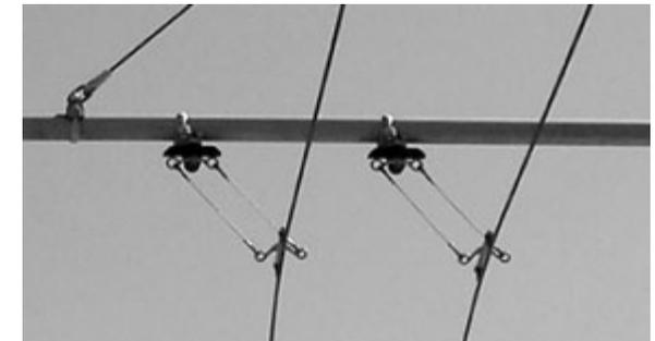
Fig. 10. The vertical elements were specifically designed for Castellón and hold the lighting system and the catenary
