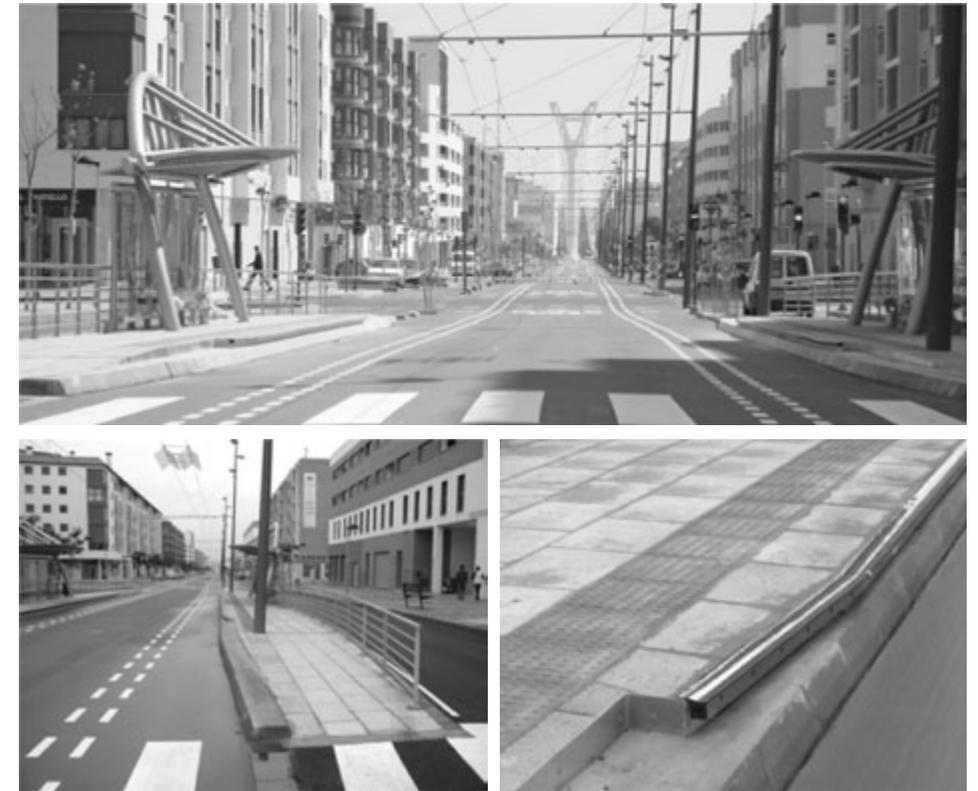
*Fig. 7 and 8. In Castellón a particular concrete kerb was designed to help the guidance system align the vehicles to the stops
