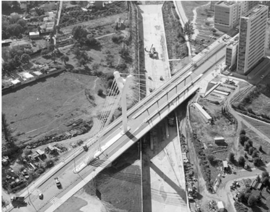
*Fig. 15. The new bridge over the “Seco” (dry) river was also design in an attempt to benefit sustainable means of transportation: wide sidewalks, cycle path, only one lane per direction for cars*
