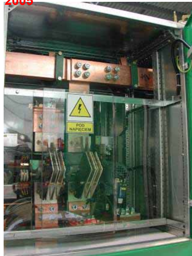
Disconnecter 2pole type STOL in rectifier cell, Motor drive
