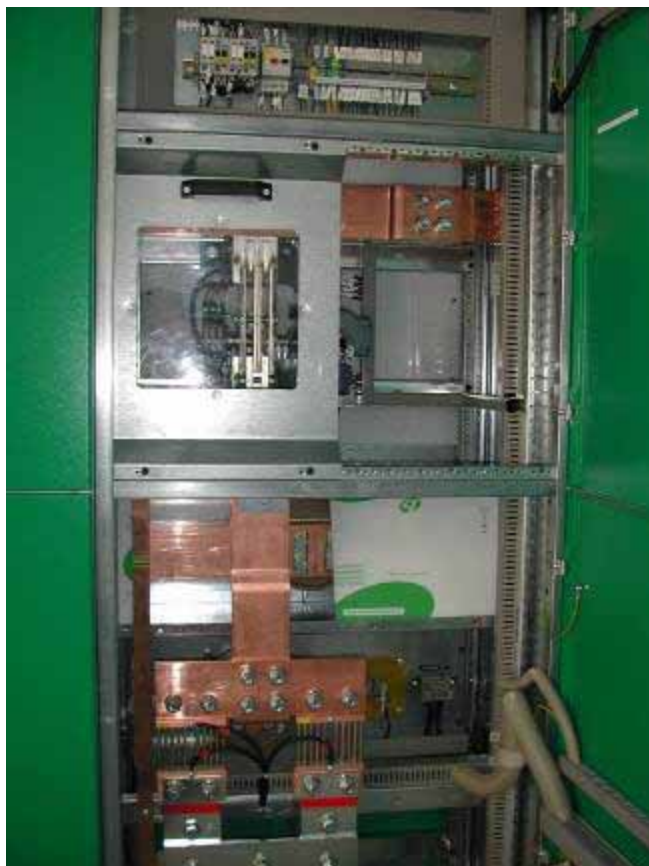
Disconnecter 1pole by-pas type STOL in feeder cell, Motor drive
